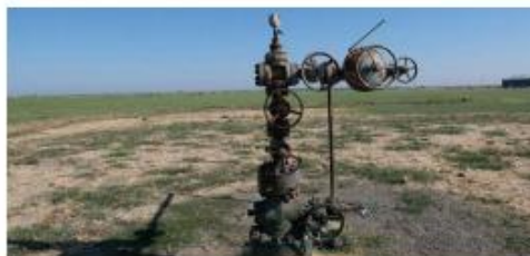
Example of an Abandoned well with pump still intact
