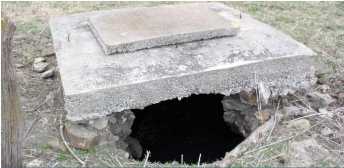
Example of an uncovered Abandoned well
